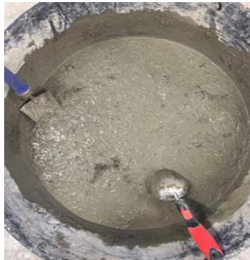
1. Mix fiber concrete
